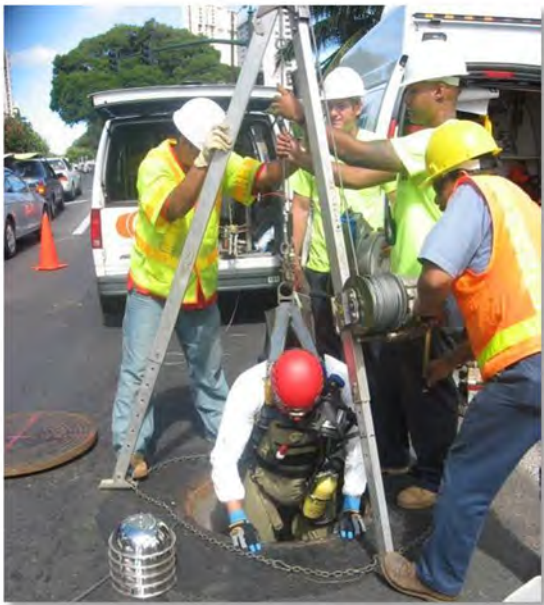
Photo 2-1. Confined Space Entry
