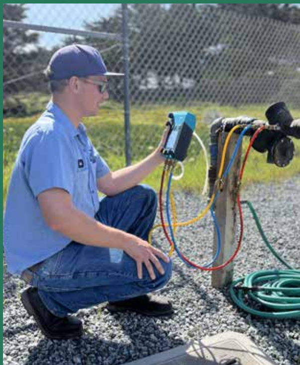
(Left) Operator exercising generator to ensure uninterrupted service during a power outage. (Above) Operator testing backflow device to ensure proper function.
