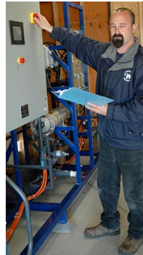
Disinfection treatment ensures safe water.
