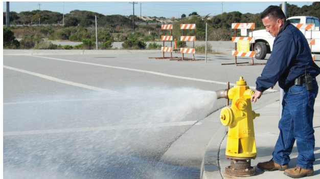
Jose Rodriguez flushes a fire hydrant to ensure water quality for customers.
