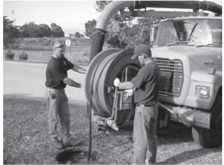
Mark Duplissie and Richard Green maintain the District's sewer lines.
