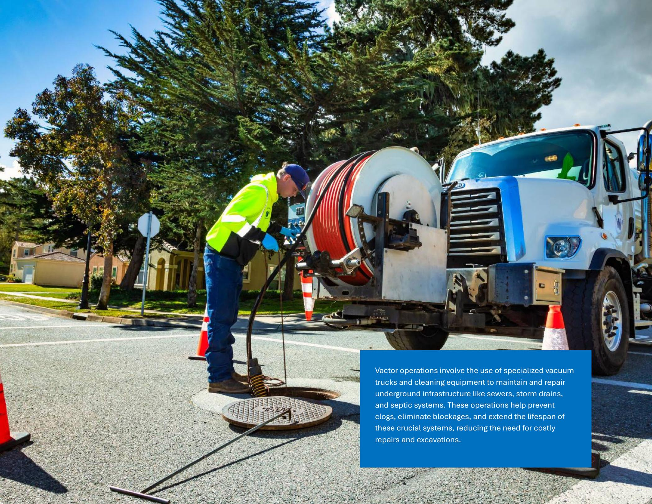
Factor operations involve the use of specialized vacuum trucks and cleaning equipment to maintain and repair underground infrastructure like sewers, storm drains, and septic systems. These operations help prevent clogs, eliminate blockages, and extend the lifespan of these crucial systems, reducing the need for costly repairs and excavations.
