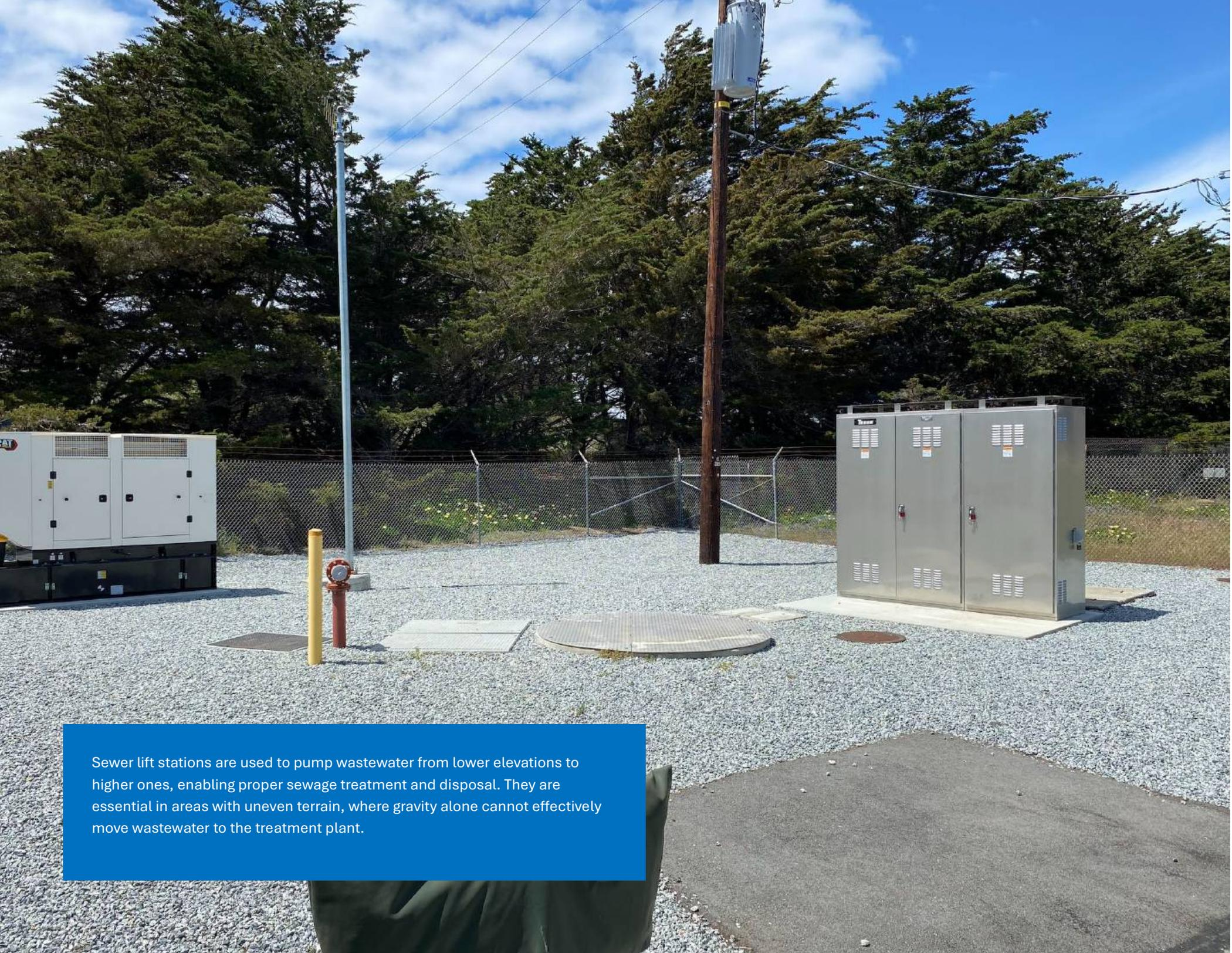
Sewer lift stations are used to pump wastewater from lower elevations to higher ones, enabling proper sewage treatment and disposal. They are essential in areas with uneven terrain, where gravity alone cannot effectively move wastewater to the treatment plant.
