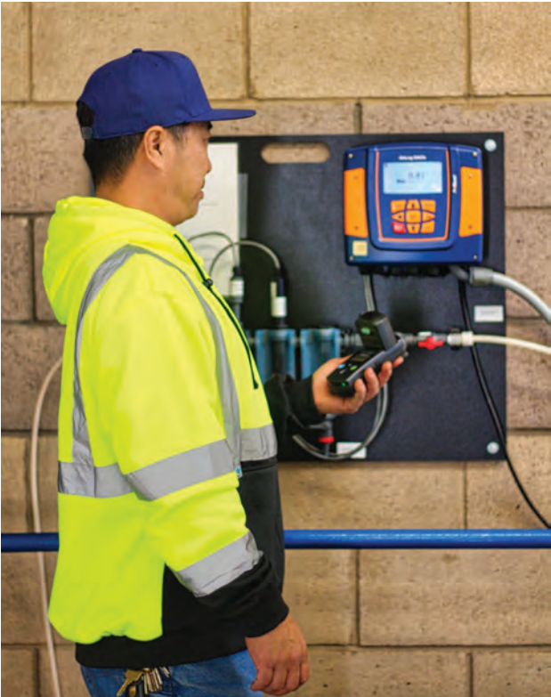
(Left) MCWD Operator exercising a water main valve to ensure proper function. (Above) MCWD Operator performing routine checks on chlorine residuals in the distribution system.
