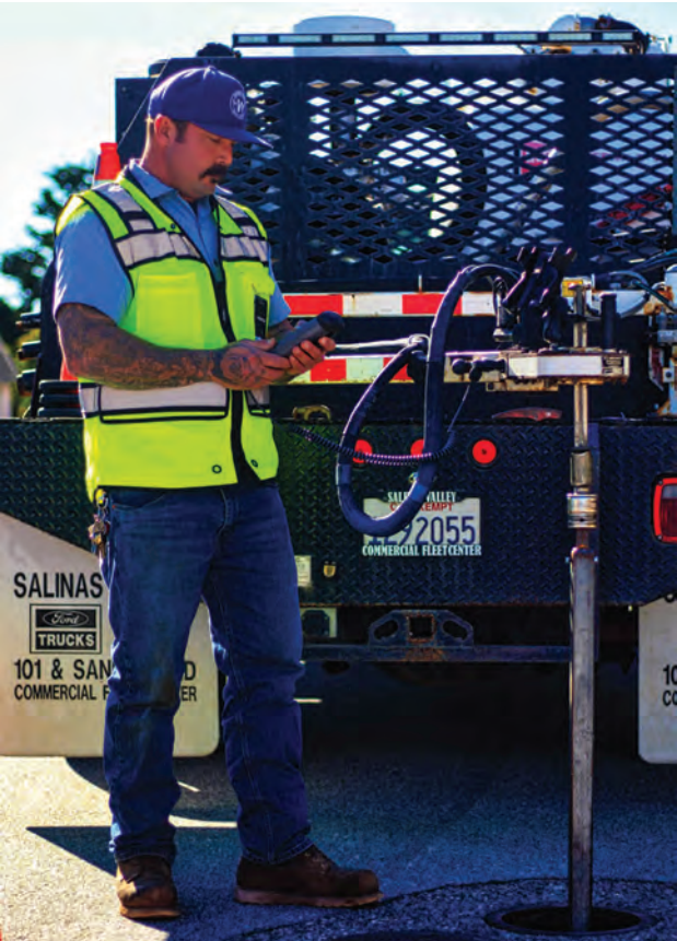
(Left) MCWD Operator exercising a water main valve to ensure proper function. (Above) MCWD Operator performing routine checks on chlorine residuals in the distribution system.
