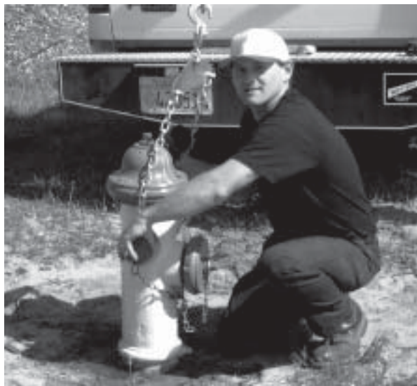
MCWD Distribution Operator Richard Green replaces fire hydrant.
