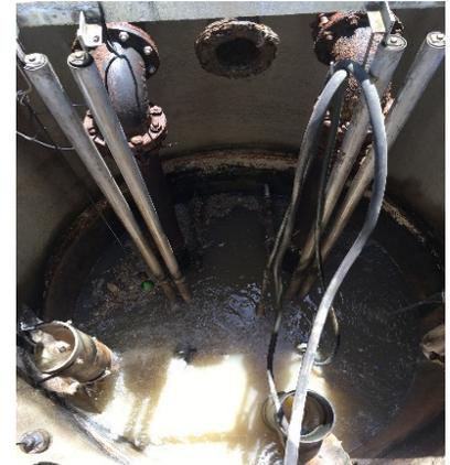
The discharge piping in the wet well shows signs of corrosion.
