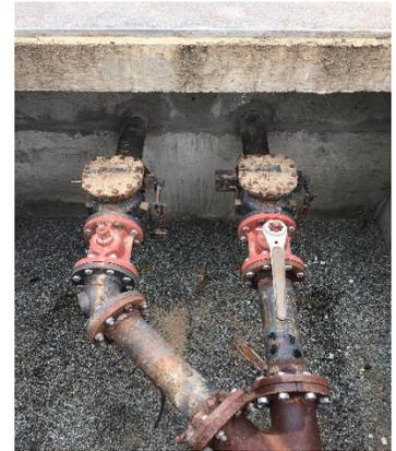
Piping and valves appear to be corroded in the Valve Vault, and are recommended for replacement.
