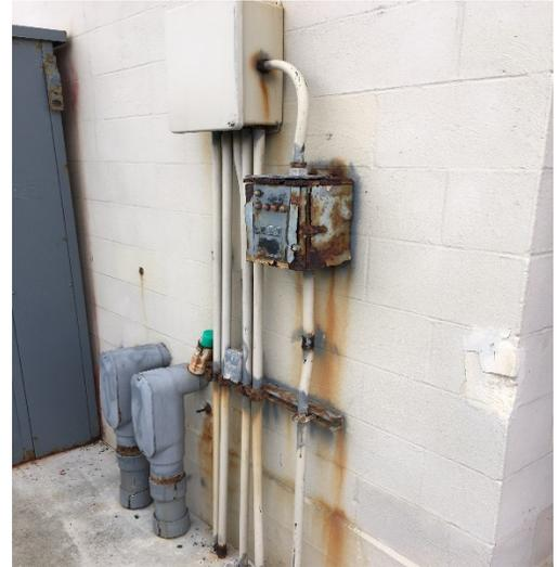
The fuel tank leak detection panel, also mounted outside, is very heavily rusted, and its functionality is in doubt. Exterior conduits and conduit supports are heavily rusted. Equipment that is mounted inside the building shows some minimal surface rust on up to 10% of the overall surface area.
