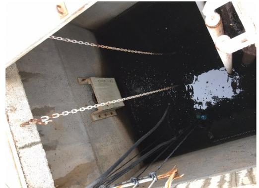
The wet well walls appear to be in good condition. The wet well dimensions are 8-ft long, 8-ft wide, and 11-ft deep.
