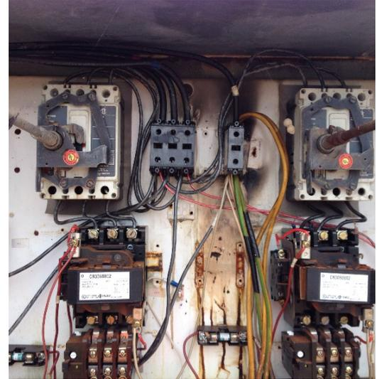
The electrical equipment consists of one cabinet with an Asco automatic transfer switch and a breaker panel, and another cabinet with pump motor starters and a Milltronics Mini-Ranger level controller. The panels show some moderate rusting. The pump control panel shows evidence that the components at one time had overheated. Existing components have a light layer of rust. These components should be replaced.
