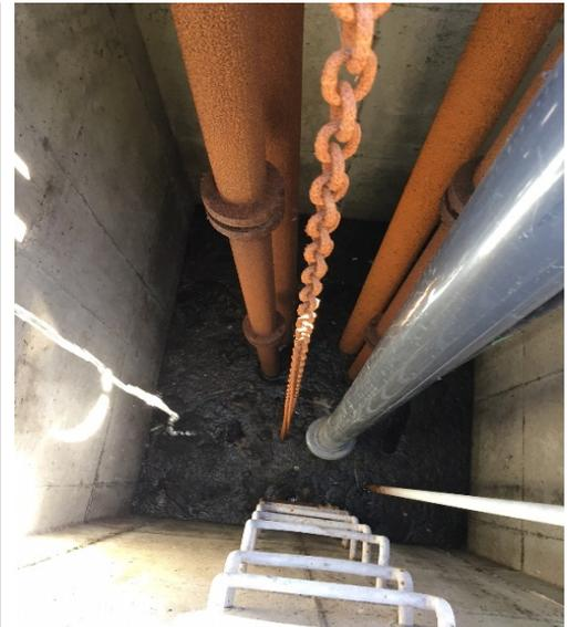
Piping and valves show signs of corrosion both inside the well and on the discharge side (For Photo - See Bypass Pump in Section 4.4.1.) of the pump station.
