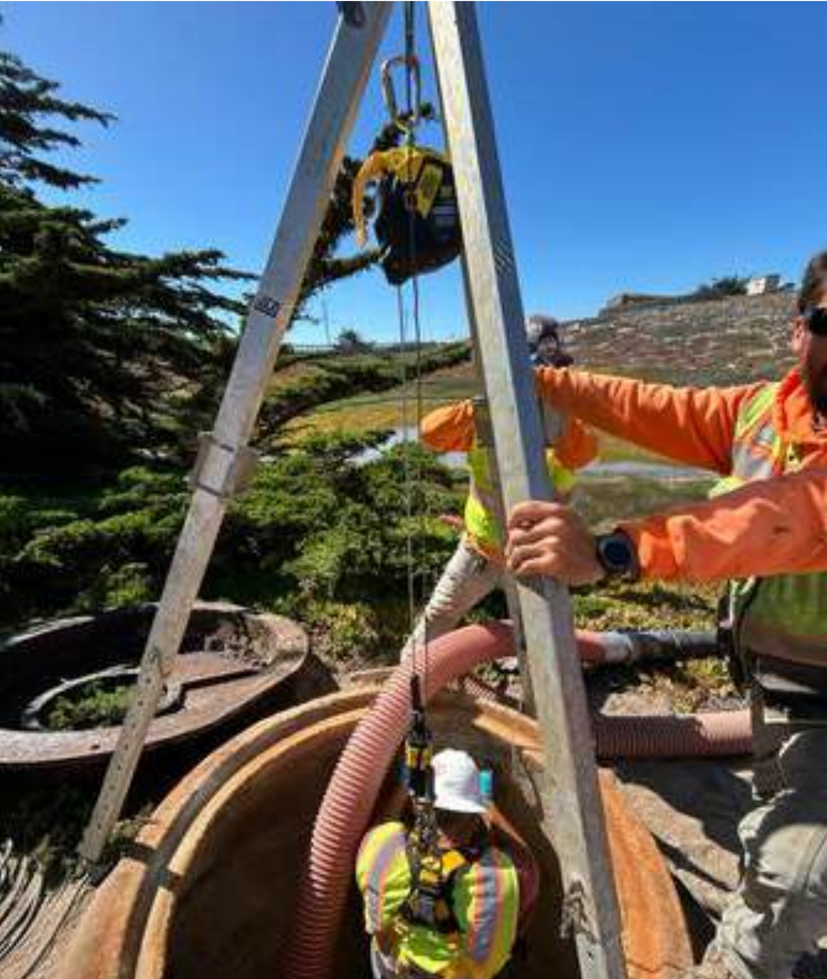
Manhole repair project—improving system safety and reliability of the wastewater infrastructure.
