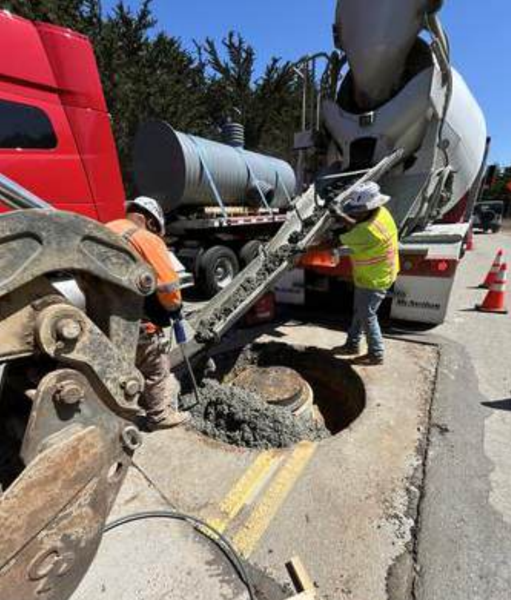
Manhole repair—restoring structural integrity and ensuring safe, reliable wastewater system access.
