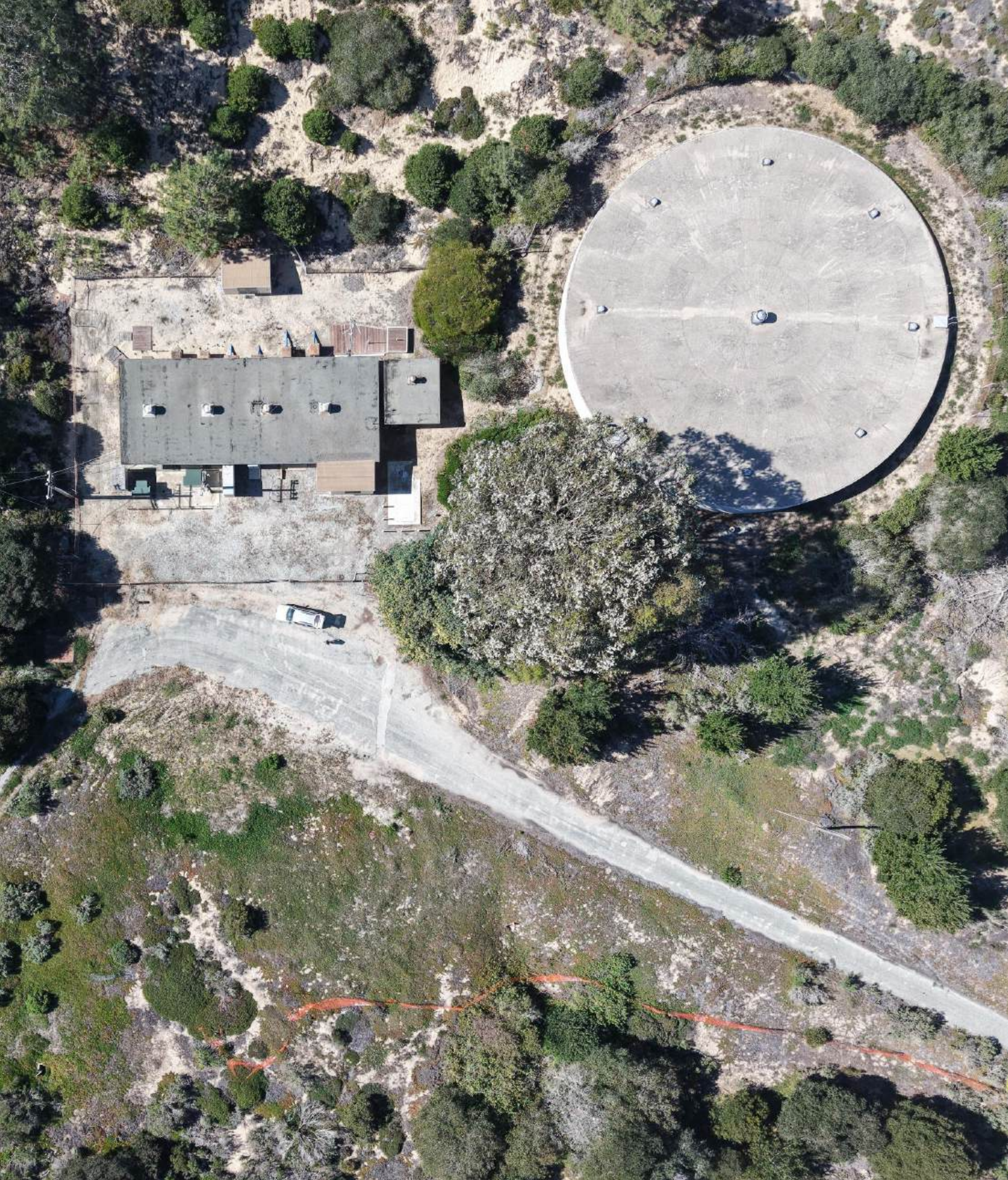
Capital Improvement Program (CIP)—investing in critical infrastructure upgrades to ensure long-term reliability and system performance.
