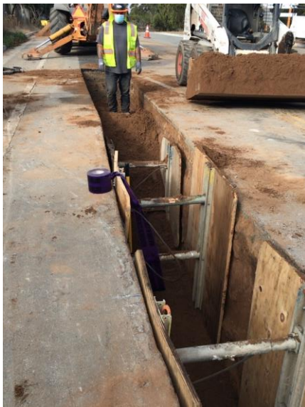
Trench shoring for pipe installation
