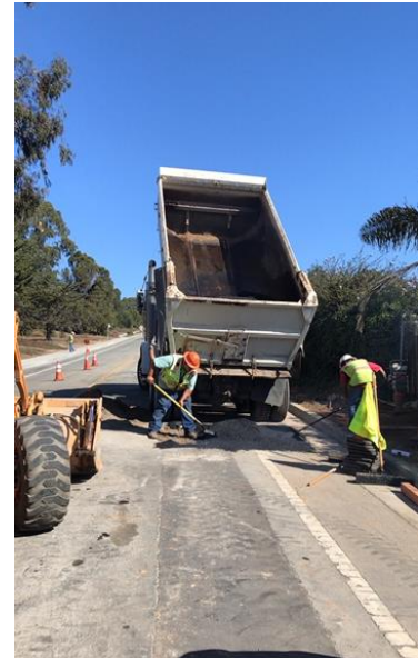
Temporary trench paving on Coe Ave
