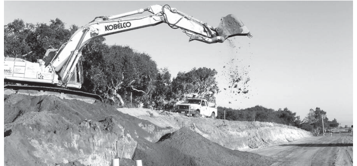
General Jim Moore Boulevard Waterline
